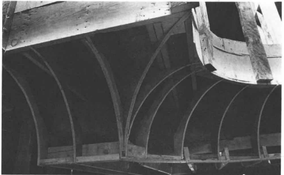
Elliptical corner braces (below) for a radiused cove ceiling can be drawn with a square and scribing rod. Both inside and outside braces are double-beveled (above) to hold intersecting pieces of lath.
